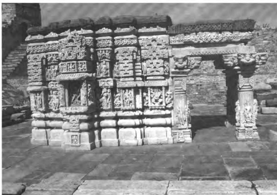
123 Temple No. 2, facing west, probably dedicated to Sadyōjāta, Survaya, dist. Shivpuri, M.P. P. 145 (Photo R.N.)
