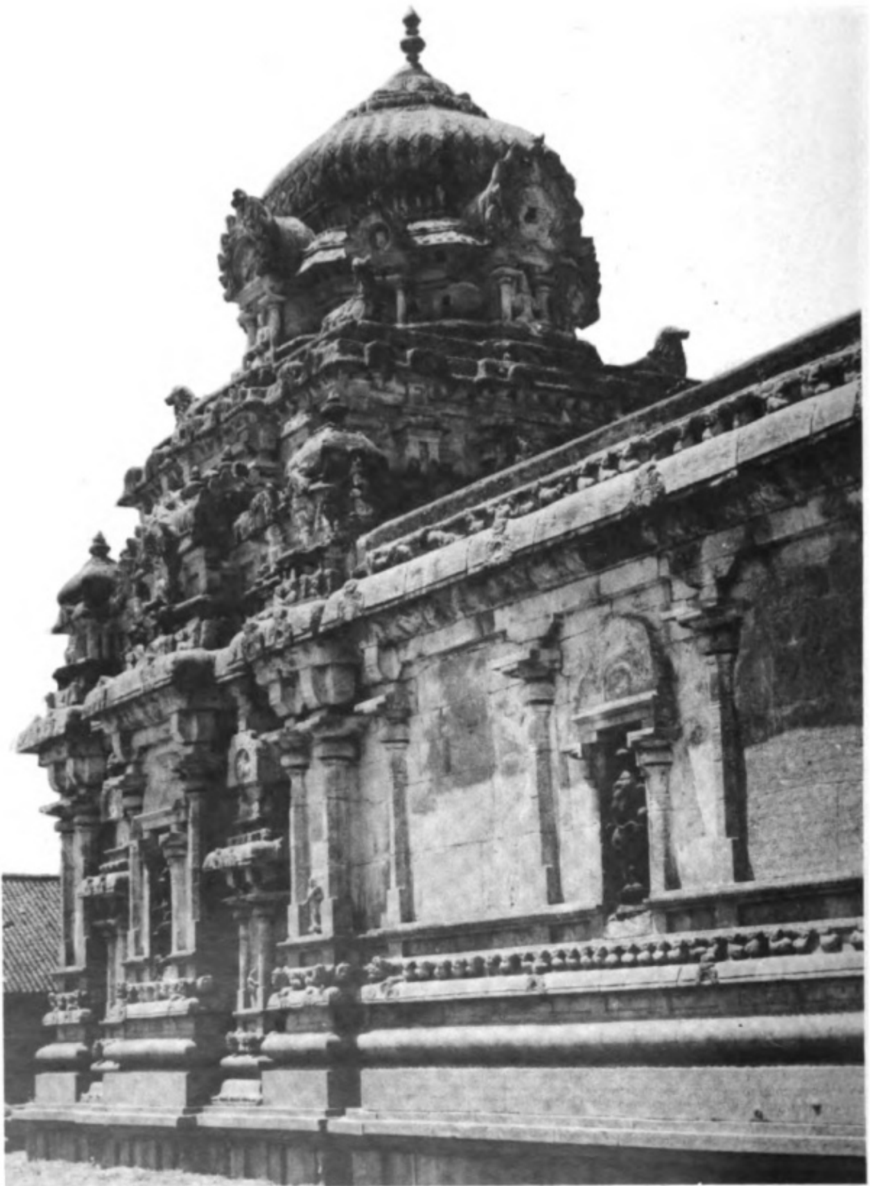
38. DADAPURAM, Manikkesvarar temple (general view)
